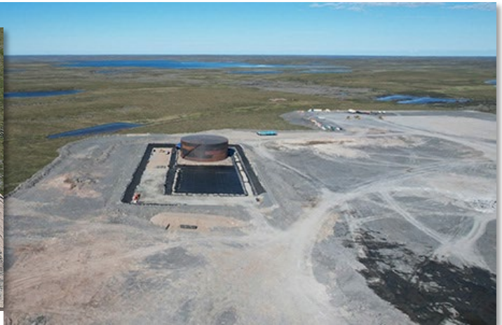
10M Liter Fuel Tank and Berm and plant/accommodation pad construction
