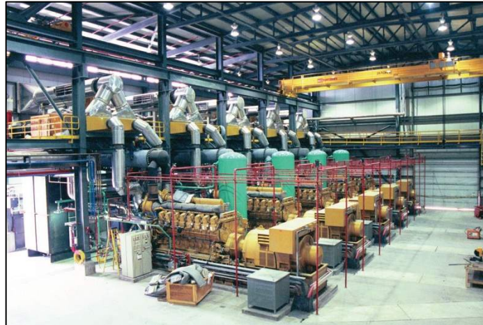
Heat recovery on diesel powerplants
