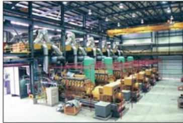
Heat recovery on diesel powerplants
