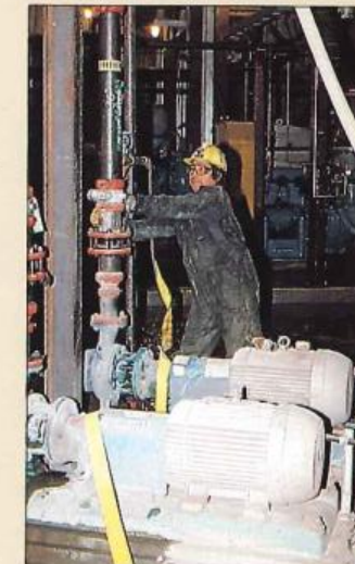
▲ Mill maintenance. ▲ Remote Controlled Scoop Tram, Nerco-Con Mine.
