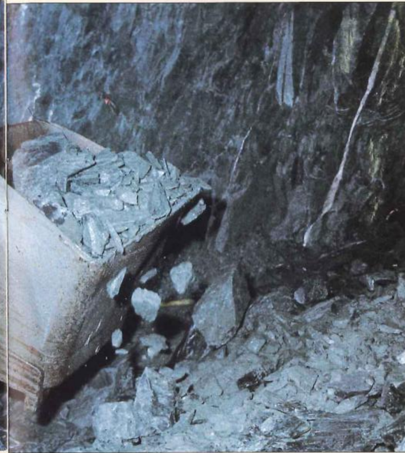
▲ A track mounted mucking machine.
