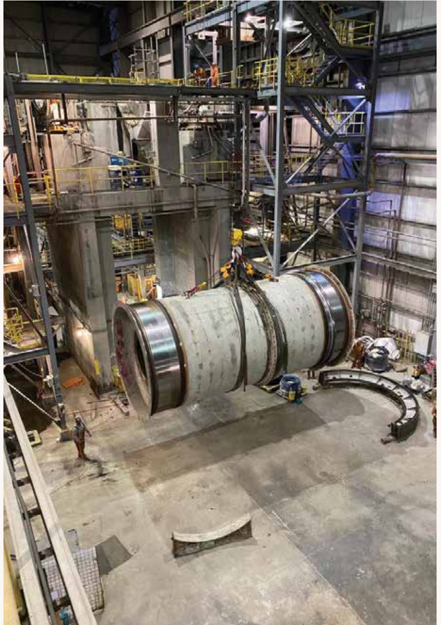
Lifting the rotary scrubber shell out of the process plant at Snap Lake.
