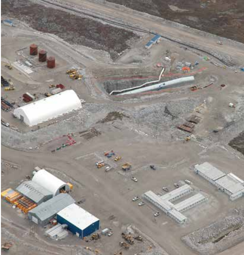
Underground mine main decline construction begins
