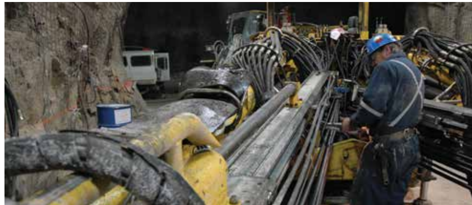
Underground hydrogeological pump test of Dewey's Fault
