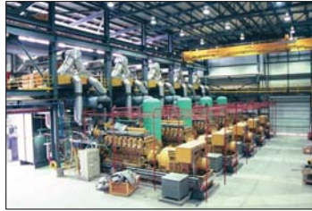
Heat recovery on Diavik diesels
