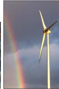
Diavik wind turbines © ENERCON GmbH
