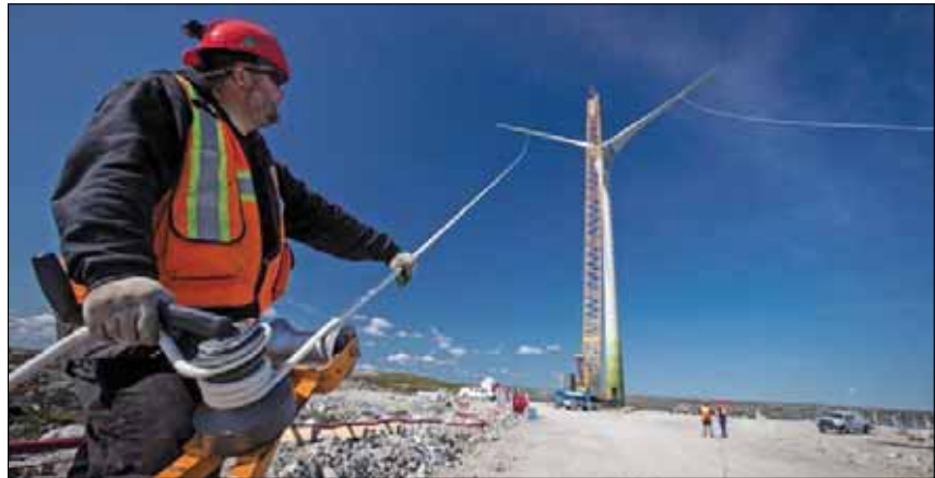
A worker feeds a support cable on one of the four 100-metre wind turbines at Diavik Diamond Mine.
