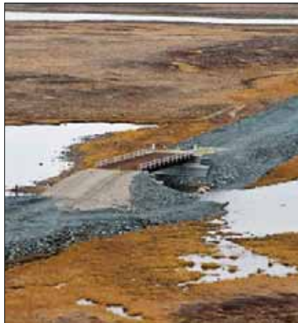
Meliadine bridge construction resulted in this river crossing over the summer.
