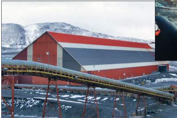
Concentrate storage facility, Nanisivik Mine, NU
