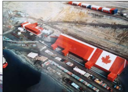
Concentrate storage facility, Polaris Mine, NU
