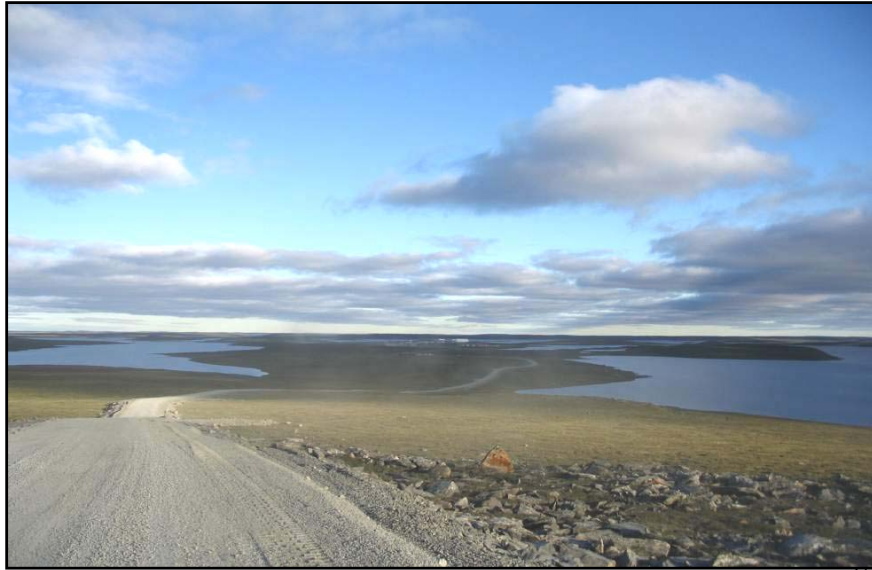
$50 million road from Meadowbank gold mine to Baker Lake, NU
