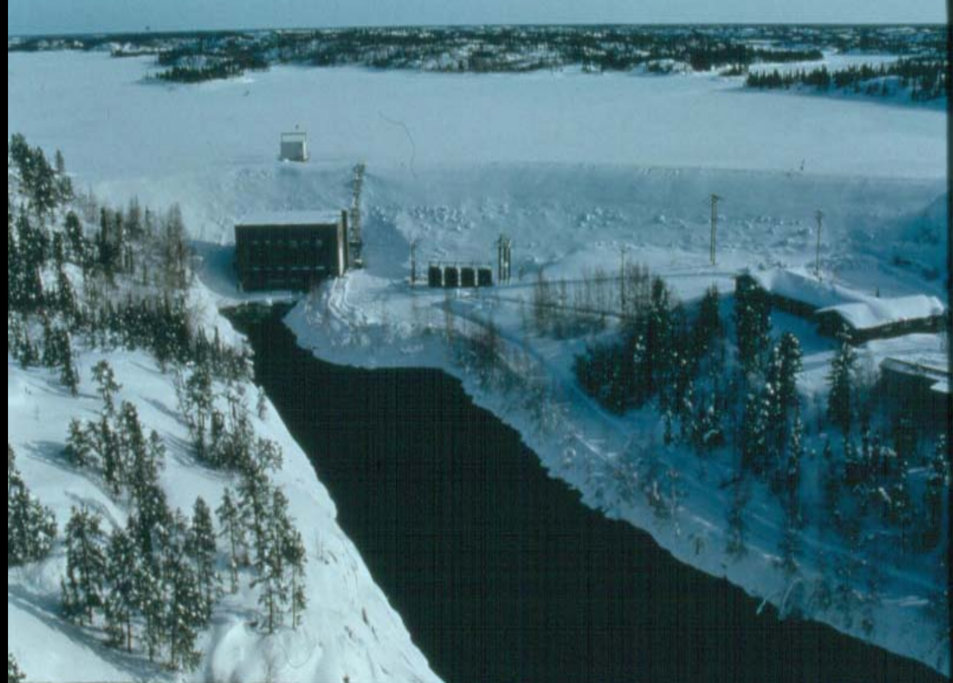
Talston River Hydro Dam – Pine Point Mine
