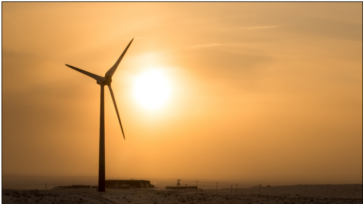
Diavik's 4 wind turbines netted them an international award in the category of BEST USE OF WIND IN MINING < 50 MW. Avalon Advanced Materials also received an award in the category of BEST USE OF RENEWABLES FOR MINE EXPLORATION at their Nechalacho project in NWT.
