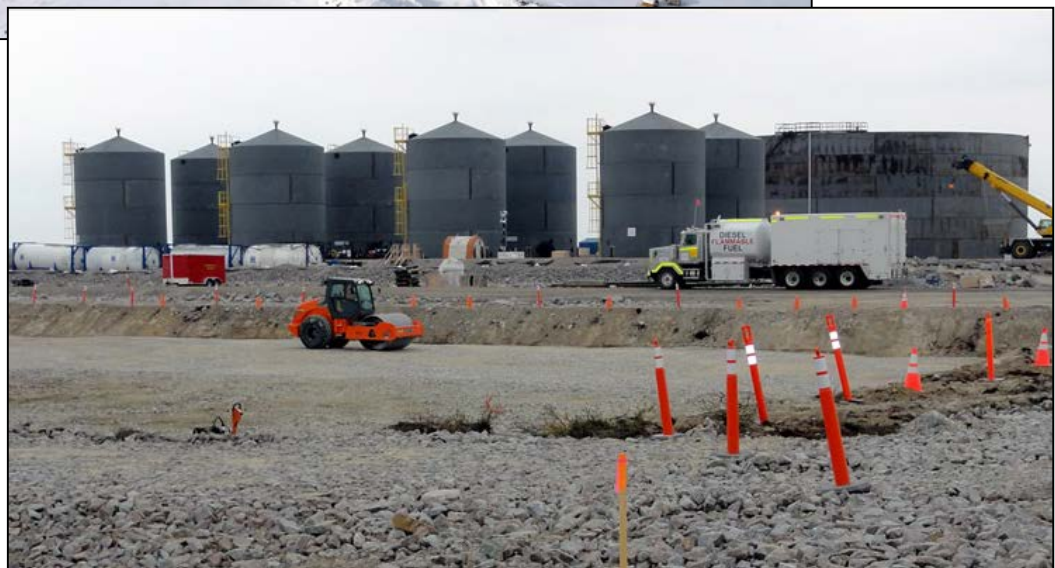
Construction progressing at the NWT's newest diamond mine, Gahcho Kué.
