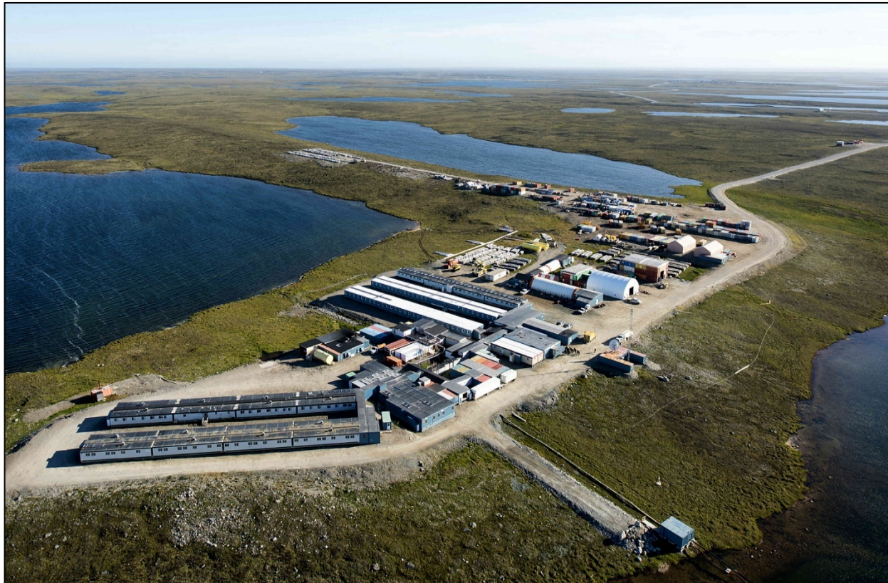
Agnico Eagle's Meliadine Project is on track to start mining in 2019. Photo: Agnico Eagle Mines
