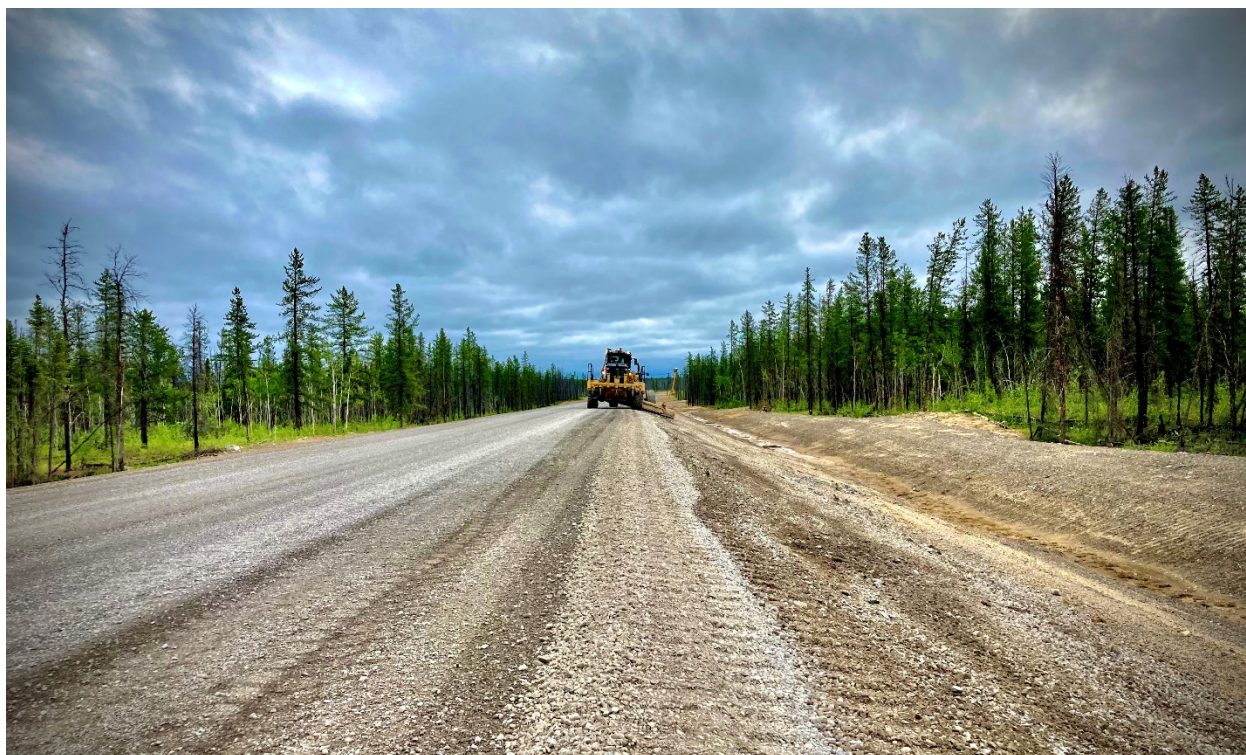
Grader finishing the roadway surface of the Tliche Highway, which opened officially on November 30. (Credit GNWT-Infrastructure)
