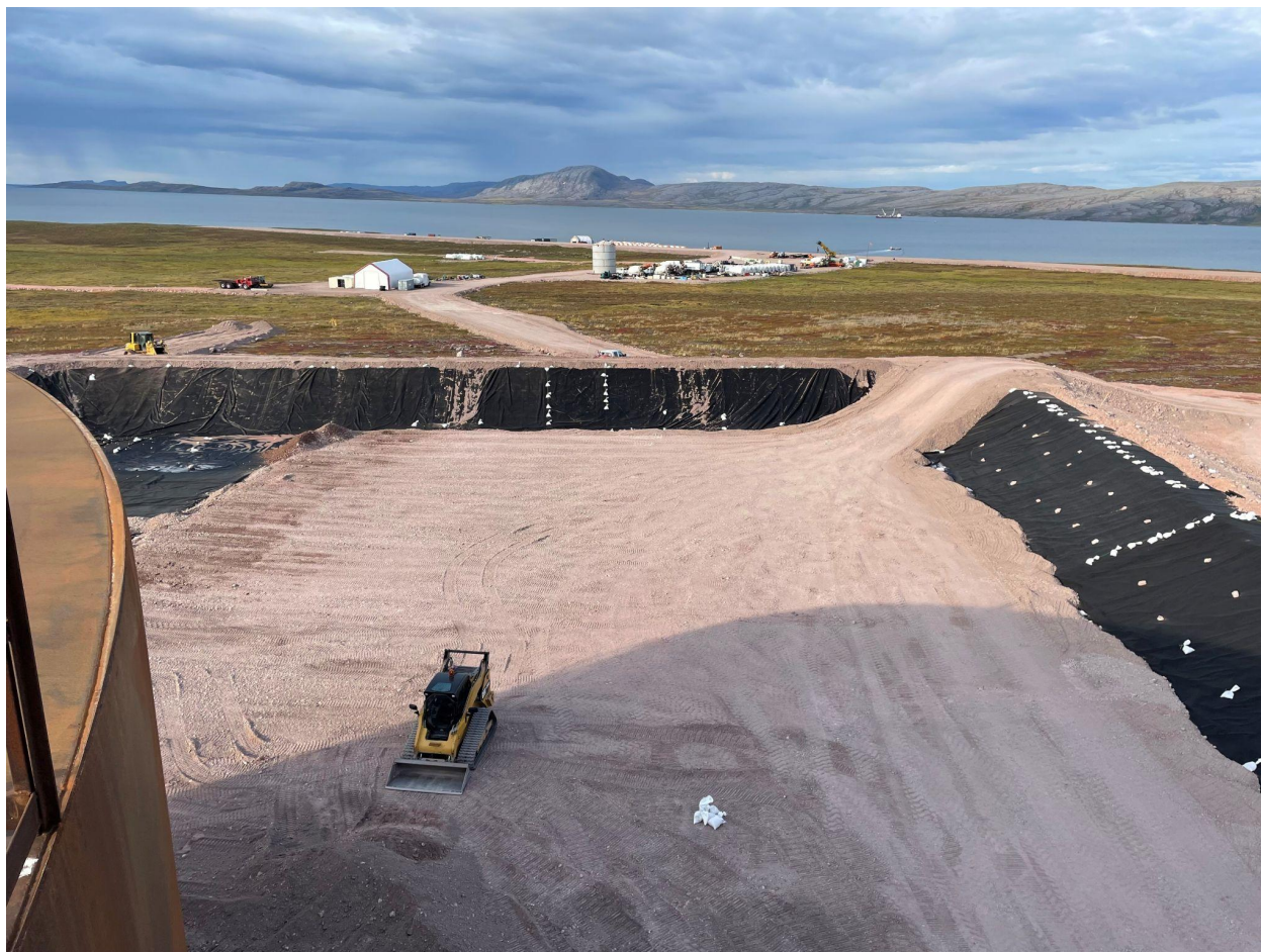
Biggest sealift for Sabina has begun. Here fuel berm with liner for 10M litre tank at the Marine Laydown Area, Bathurst Inlet, Arctic Ocean.
