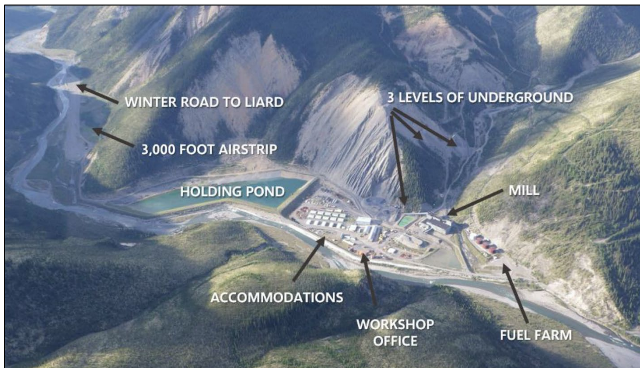
Prairie Creek mine site facilities. (from NorZinc Corporate Presentation, March 2021)
