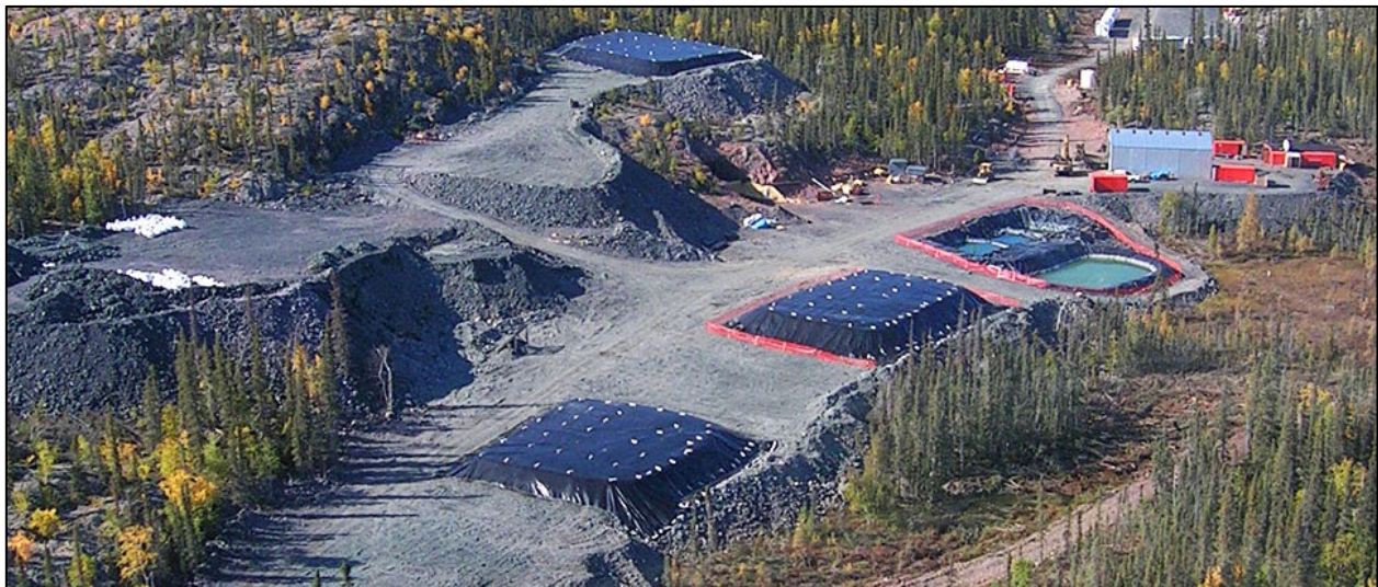
Aerial view of NICO site during test mining. Fortune Minerals photo
