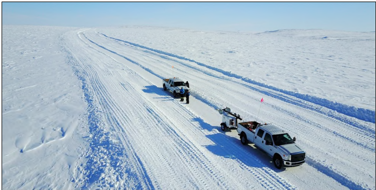
In 2019, Sabina's new winter road broke trail from the Bathurst Inlet marine laydown area to the site of the future Back River mine. Sabina photo
