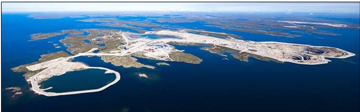
Aerial view of the A21 dike in 2017 before it was sealed and the water behind it pumped out to allow open pit mining. Note the other two dikes surrounding open pits to the right. The first of these was awarded Canada's highest engineering honours for its innovative and safe design. Photo courtesy Rio Tinto
