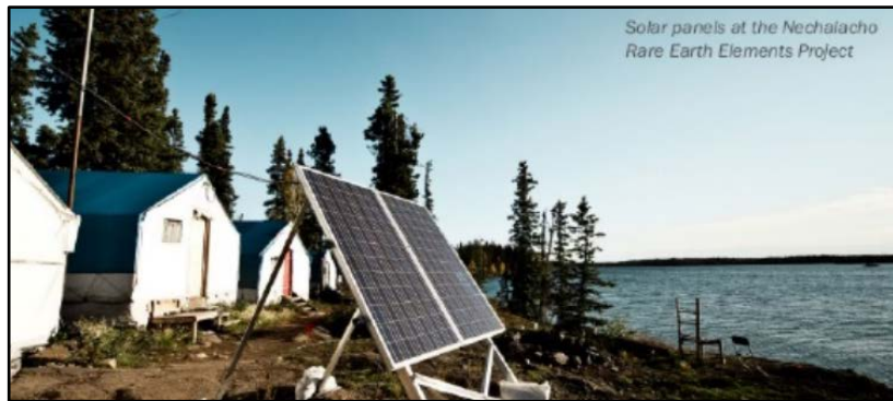
Solar panels at the Nechalacho Rare Earth Elements Project.
