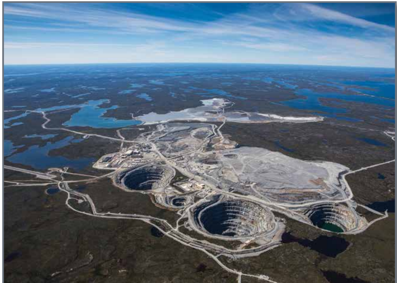
EKATI mine is Canada's first diamond mine.
