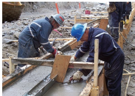
Laying forms at Diavik Diamond Mine. Photocredit: Kitikmeot Corporation and Jiri Hermann.
