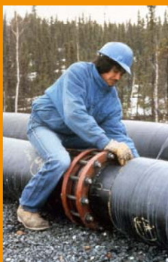
Tlich workers at Colomac Mine, 1990
