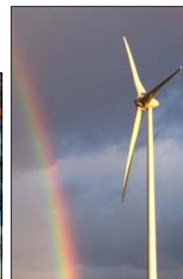
Diavik wind turbines © ENERCON GmbH
