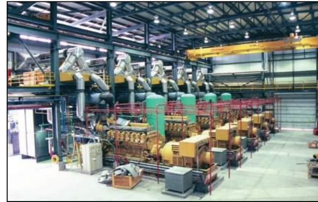
Heat recovery on diesel electrical power plants
