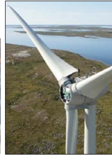
Diavik wind turbines
