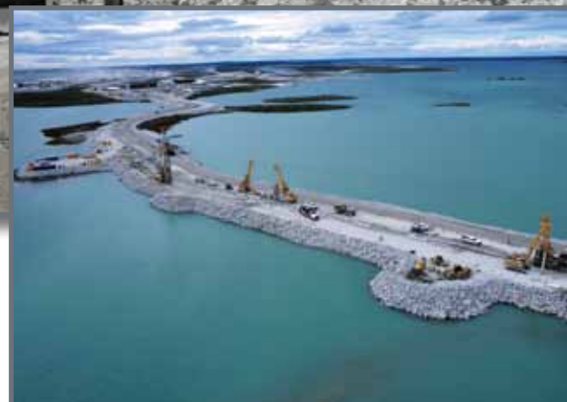
Construction of the first dike at the Diavik mine
