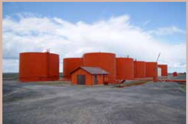
Tank farm Lupin Mine Courtesy of AANDC
