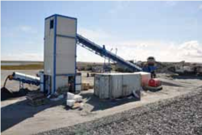
Sampling tower, Meliadine project Courtesy of Agnico-Eagle Mines Limited
