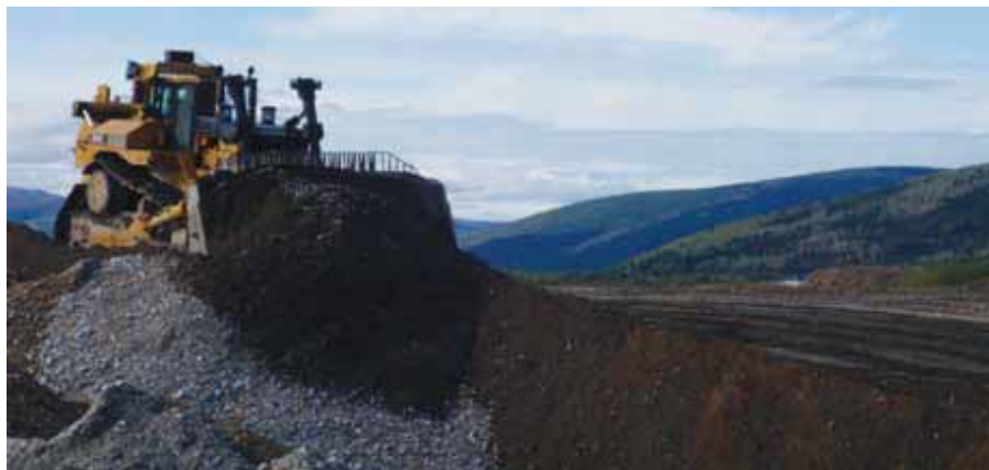
A dozer carries out reclamation work. Photo courtesy of Cobalt Construction.
